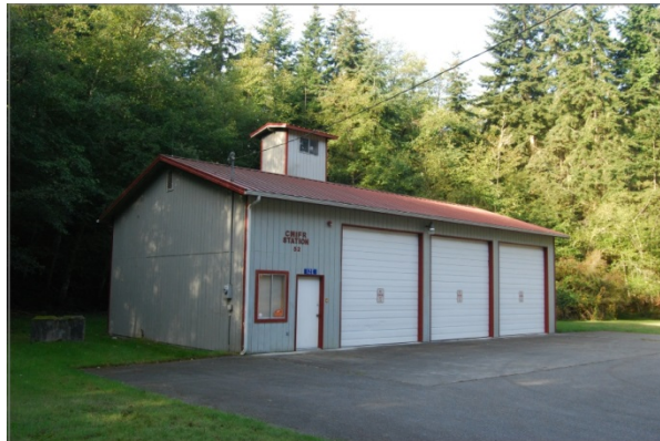
Figure 8. Station 52 (Logistics Facility)
