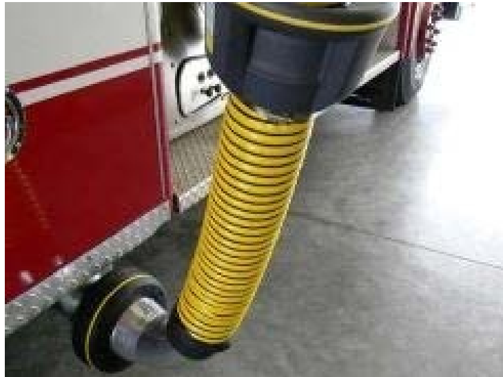
Figure 30. Exhaust Removal System
