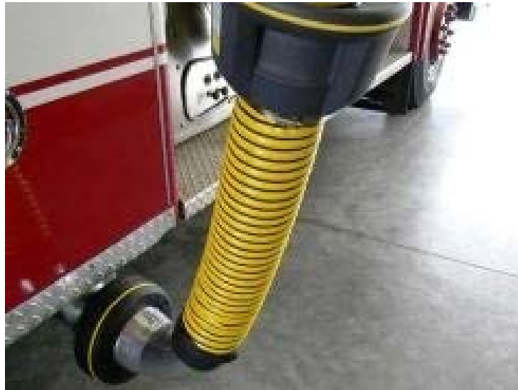
Figure 30. Exhaust Removal System
