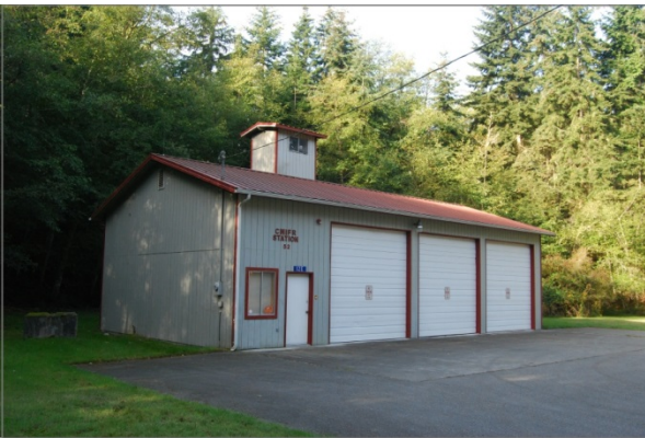
Figure 9. Station 52 (Logistics Facility)
