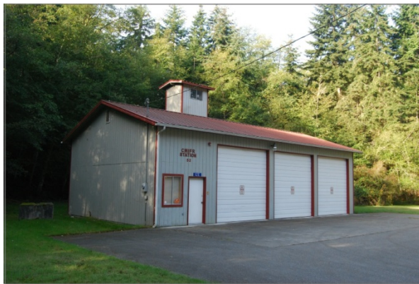
Figure 9. Station 52 (Logistics Facility)
